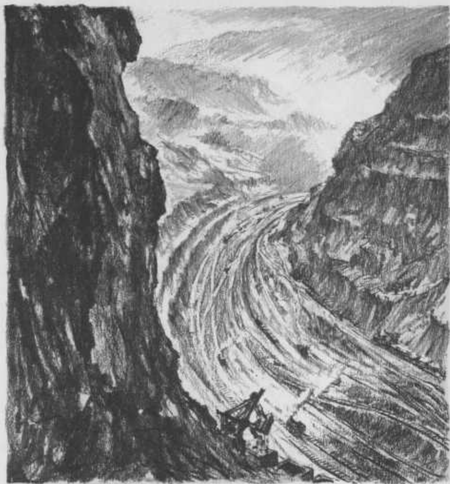
Digging the Cut
